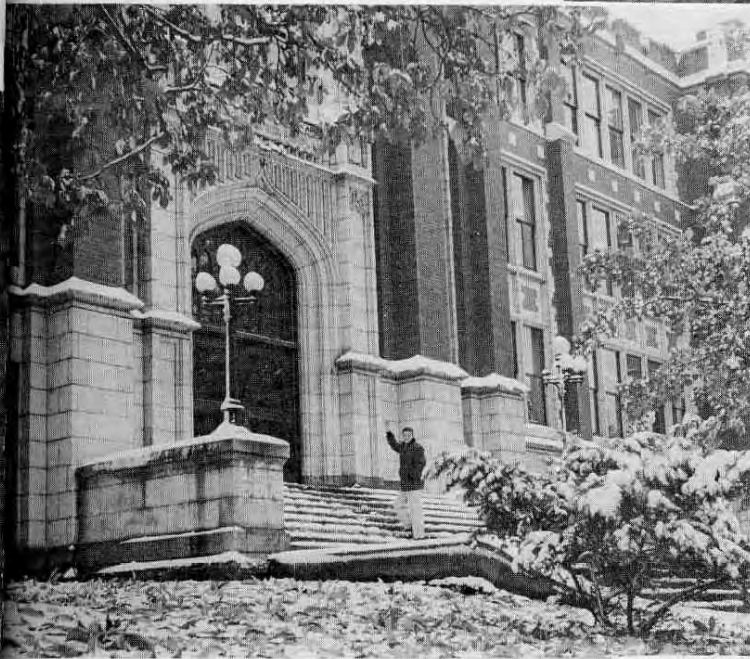
Main Entrance from East
